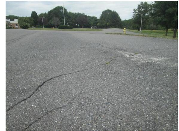
Parking spots to the south and east of the building can be replaced with porous asphalt to capture and infiltrate stormwater. A preliminary soil assessment suggests that more soil testing would be required before determining the soil's suitability for green infrastructure.
