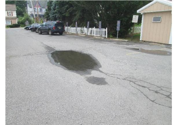
Parking spots to the north of the building can be replaced with porous asphalt to capture and infiltrate stormwater. Runoff from the roof top can be disconnected and drain into the rainwater harvesting system. A preliminary soil assessment suggests that the soils have suitable drainage characteristics for green infrastructure.
